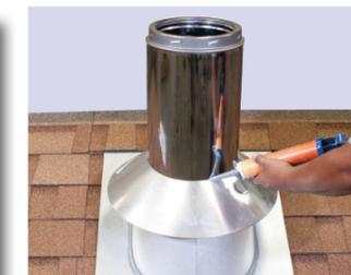
13. Slip storm collar around chimney and slide down. Apply high temperature silicone sealant where storm collar will meet chimney.
