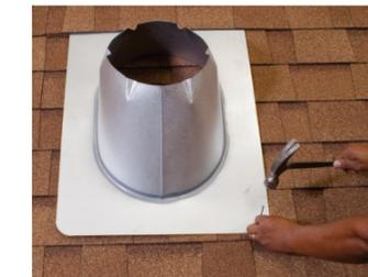
11. Slip the flashing over the roof hole so the top edge is under the shingles above. Nail the flashing to the roof across the top and down 1/2 each side. Seal flashing and nailheads with weatherizing sealant.
