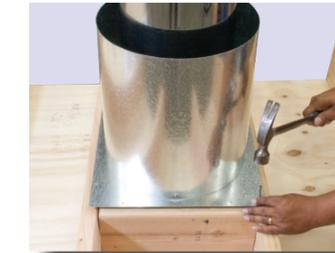
6. Slip insulation shield over chimney until base sits squarely on framed opening or nests in the support box. Nail to opening or screw to box.
