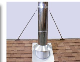
14. If the chimney extends 5' or more above the roof penetration an Extended Roof Bracket is needed.
