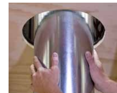
9. Hole in roof must provide at least a 2" clearance all around the chimney. Add more chimney sections, and twist to lock.
