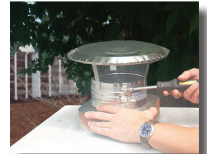
6. Trim excess liner and Top Plate, then attach Raincap.
