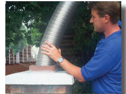
3. Insert Ventinox into chimney.
