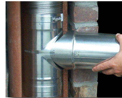
4. Feed liner through Snout's drawband, then fasten.
