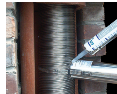
8. Fasten and seal Universal Take-off to Ventinox.
